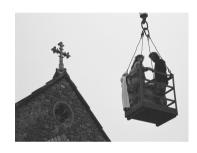
The cost to scaffold the east end to give working access to the cross was unrealistic considering the job to be done, but with some lateral thought we secured the use of a large crane from King Lifting, which appeared at 7.00am on Sunday morning 13 April. It was not the fixed platform type that Mark had expected. He was hoisted up in a swinging basket, which he had to buffer off the east gable to prevent damage to the stonework and he had to hang on whilst he worked!
